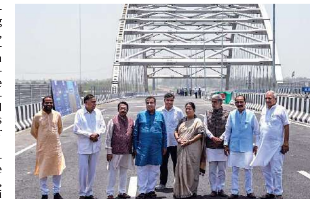
Union Minister of Road Transport and Highways Nitin Gadkari along with Chief Minister Rekha Gupta and others conduct a joint on-site inspection of the Delhi-Mumbai Expressway Link (NH-148 NA) project, New Delhi
